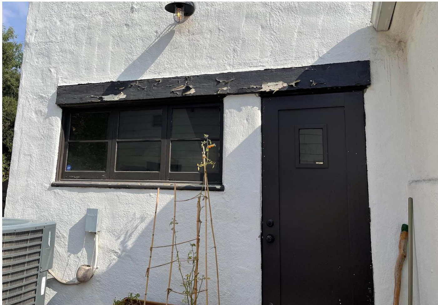
Repair and repaint window and lintel - south exterior
