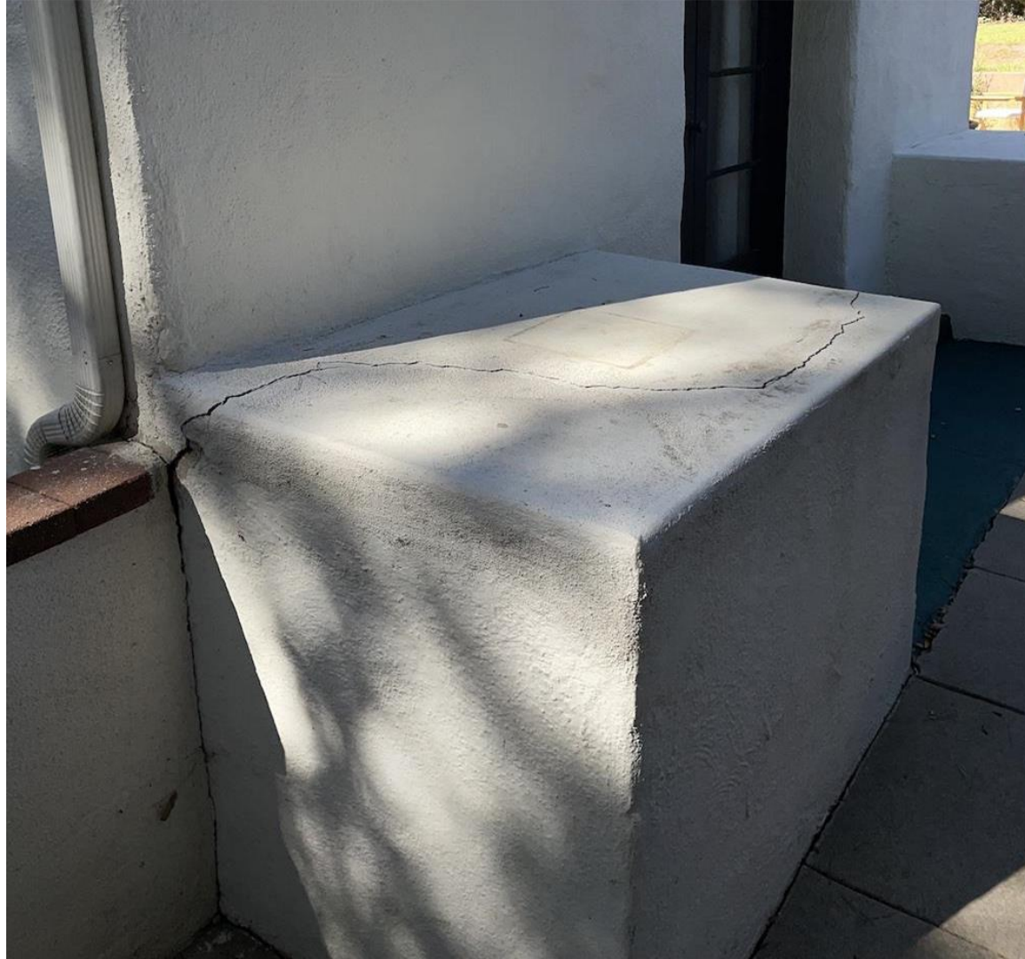
Repair crack in stucco at northeast corner of house
